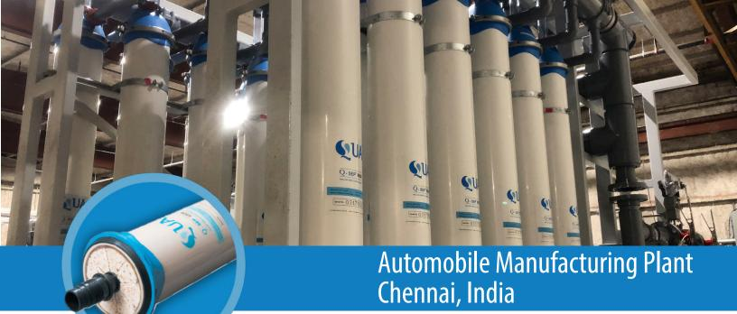
QUA's Q-SEP UF membranes replace other manufacturer's membranes to meet client's performance criteria and delivery schedule.
